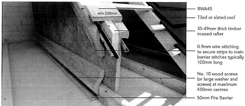
Figure 6 Half hour protection for timber truss construction 35 to 49mm thick.
